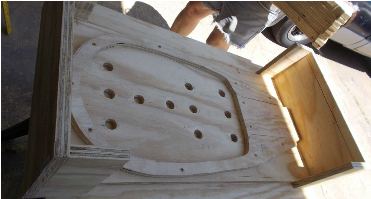
Figure 5. The completed outer securing form forms an open sided box with holes drilled into the bottom to prevent a vacuum from forming, aiding the form-removal process. The raised form on the floor of the box will form the top of the box. The innerform pieces will sit in the central area, and are secured in place by the raised area. The actual nest box is poured upside down.
